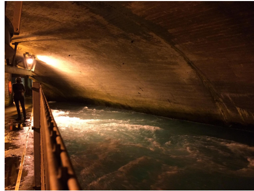
Figure 3. Inside the hydroelectric power plant
